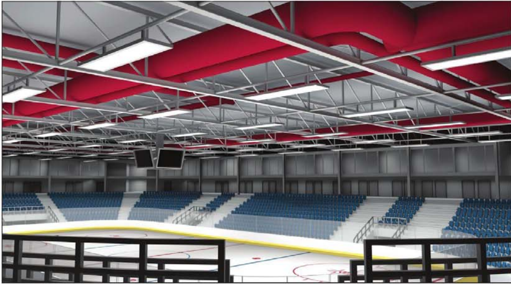
Fabric duct is ideal for sports facilities because flying objects cannot damage or dent it.
