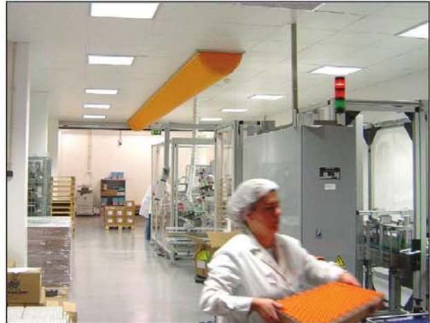
The D-shaped fabric duct distribution system is an ideal application for low clearance ceilings that cannot accommodate low hanging metal or a round fabric duct.
